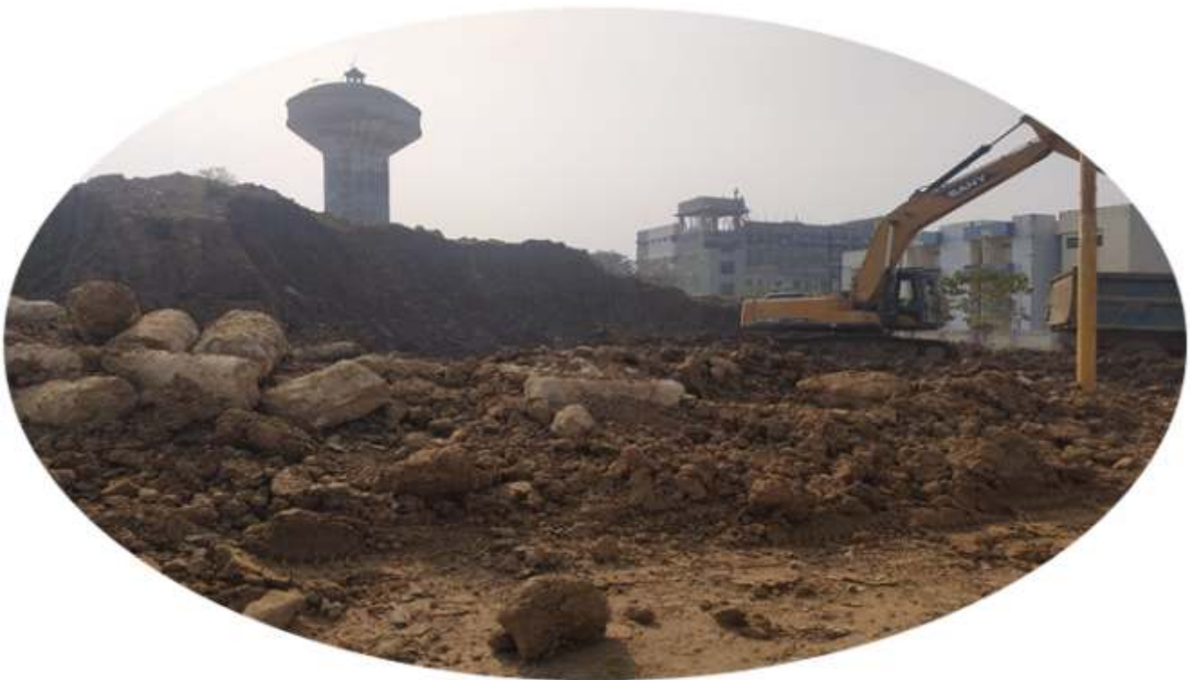
Construction of 200- Bedded RIO Building(ThroughCPWD,Patna)
