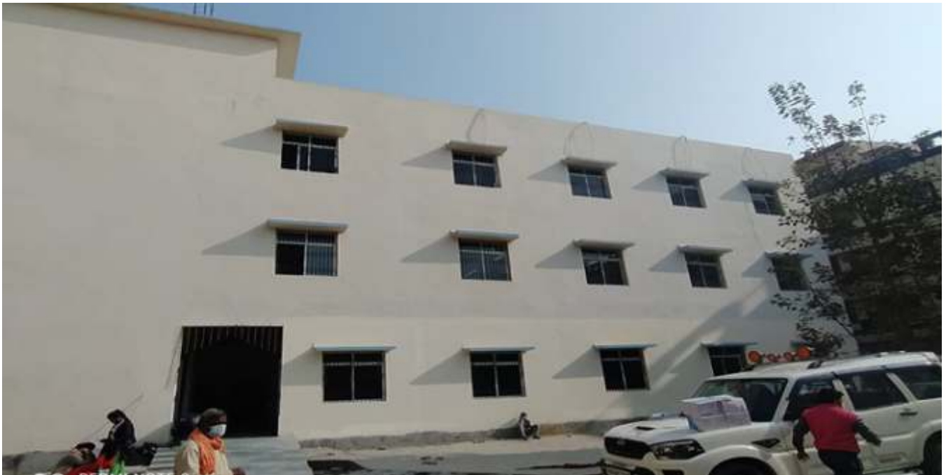
Construction of new RIO building
