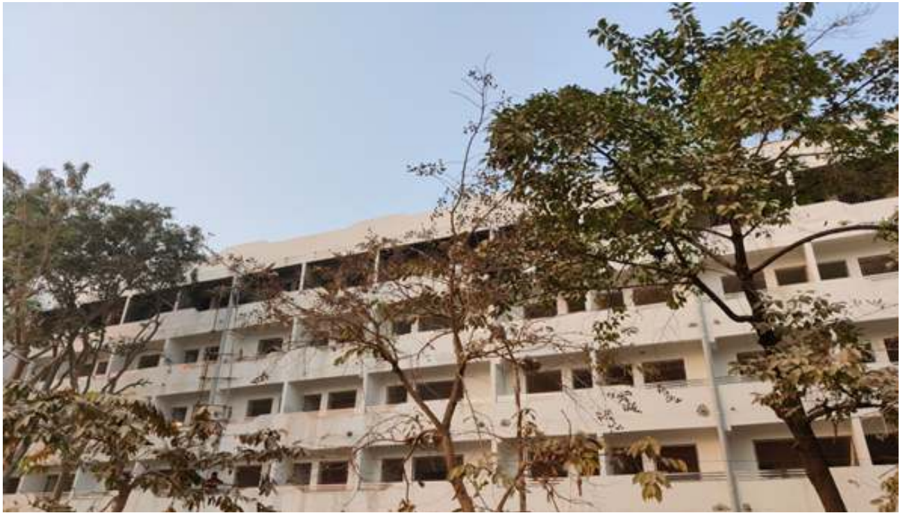
Construction of new 100 BEDED Intern Girls Hostel Building
