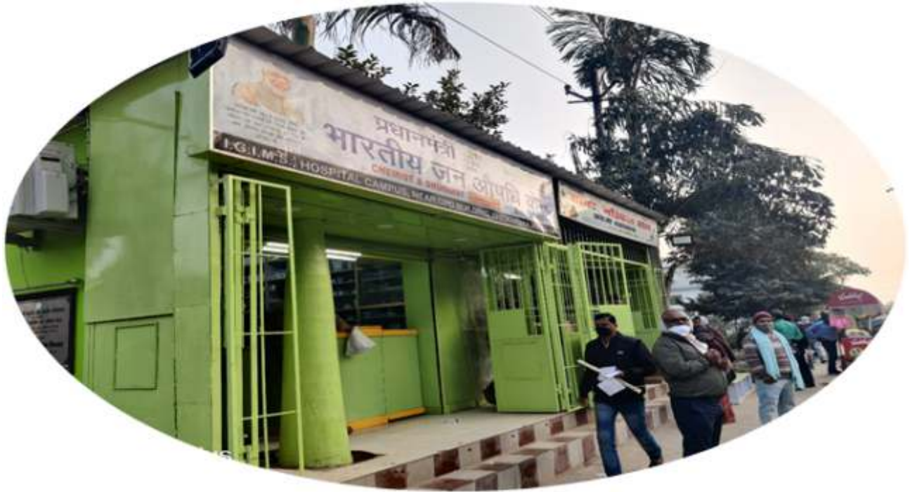
Construction of Generic Medical Shop under scheme of Pradhan Mantri Jan Anushand Kendra near OPD.
