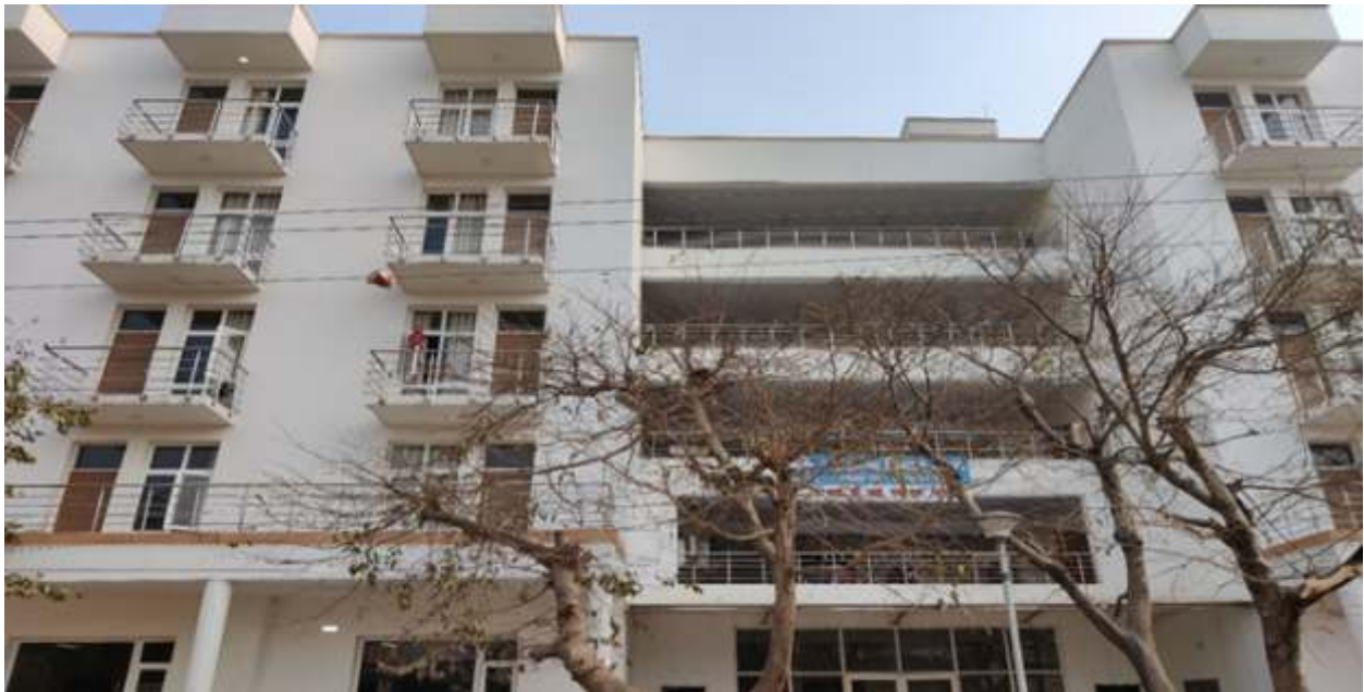
The Four Storied "Vishram Sadan" under CSR programm by M/S Power Grid Corporation
