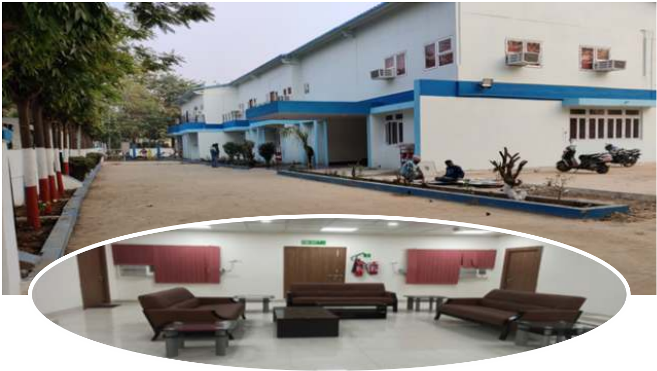
Modernization of Guest house Building.
